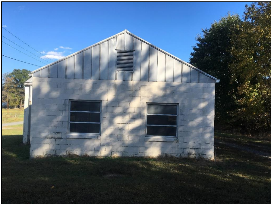
Photo 39: Building 1145, west side
