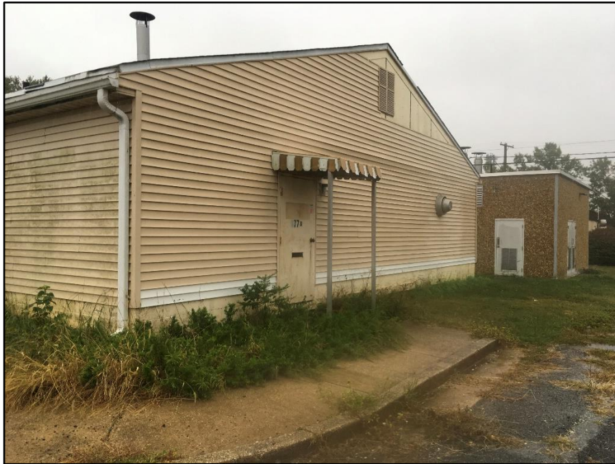
Photo 07: Building 177B, west side
