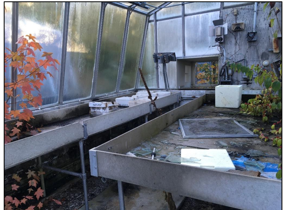
Photo 32: Buildings 470AA – 470JJ, representative photo of inside greenhouse
