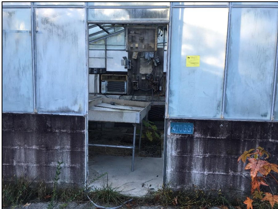
Photo 31: Building 470GG, inside
