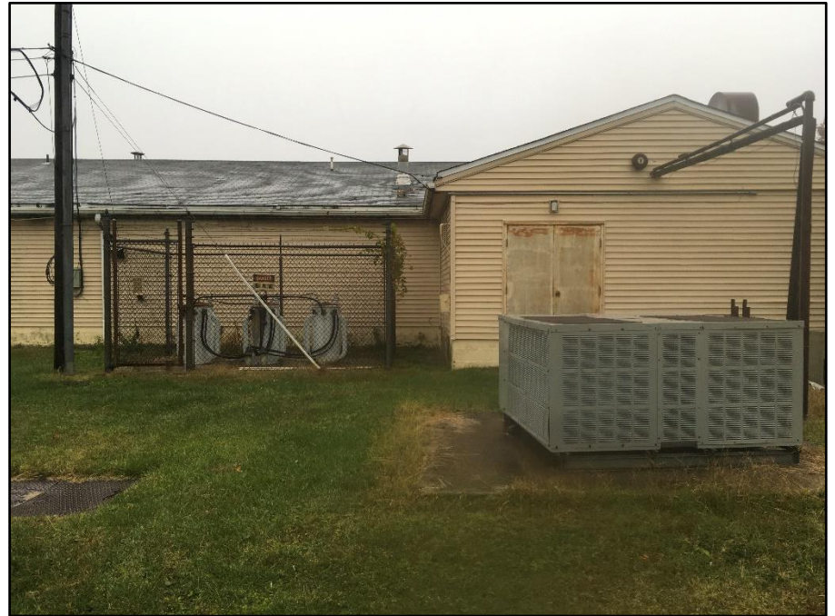
Photo 06: Building 177B, south side
