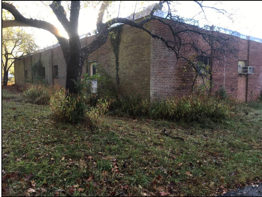
Photo 18: Building 465, north and west sides
