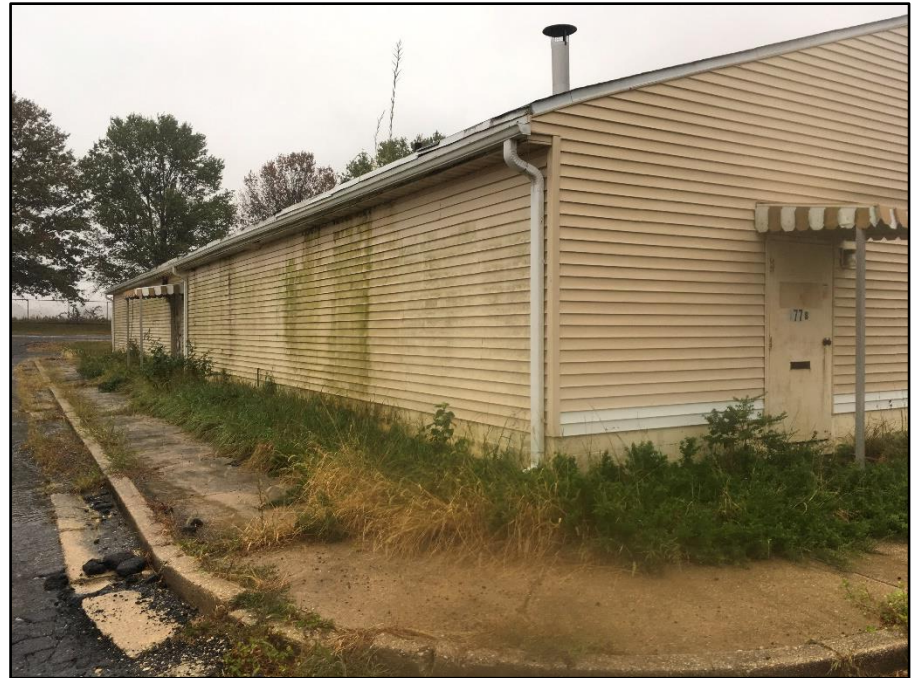
Photo 08: Building 177B, north side
