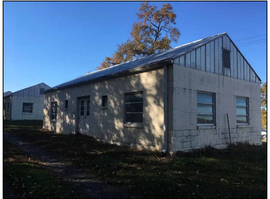
Photo 38: Building 1145, south (back) and east sides
