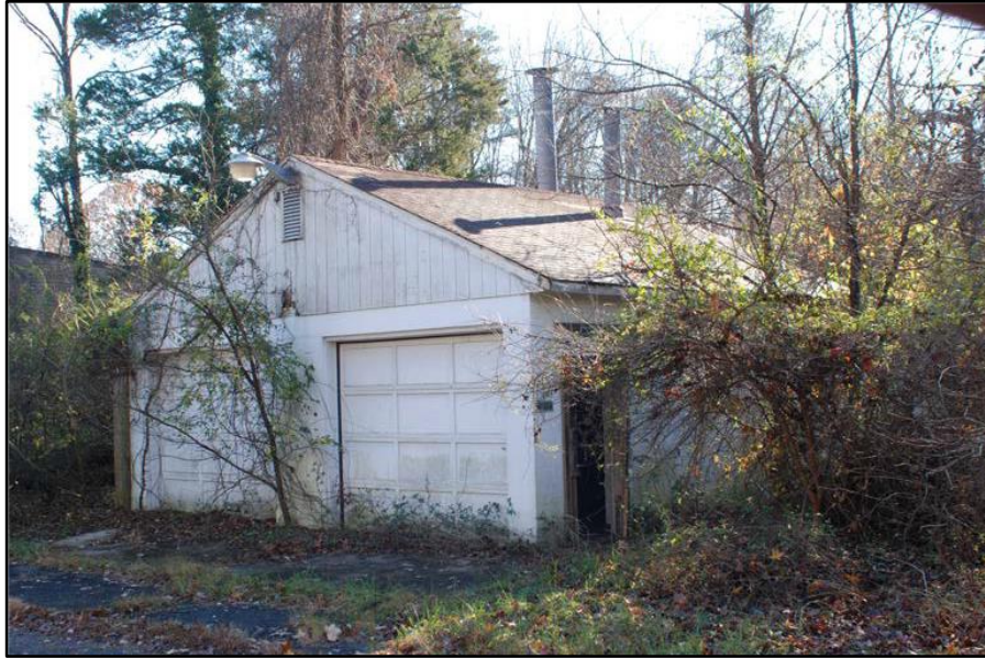
Building 288A (a)
