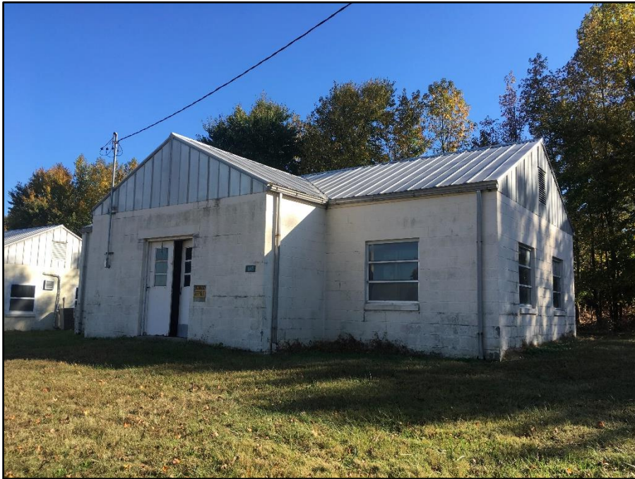
Photo 37: Building 1145, north (front) and west sides
