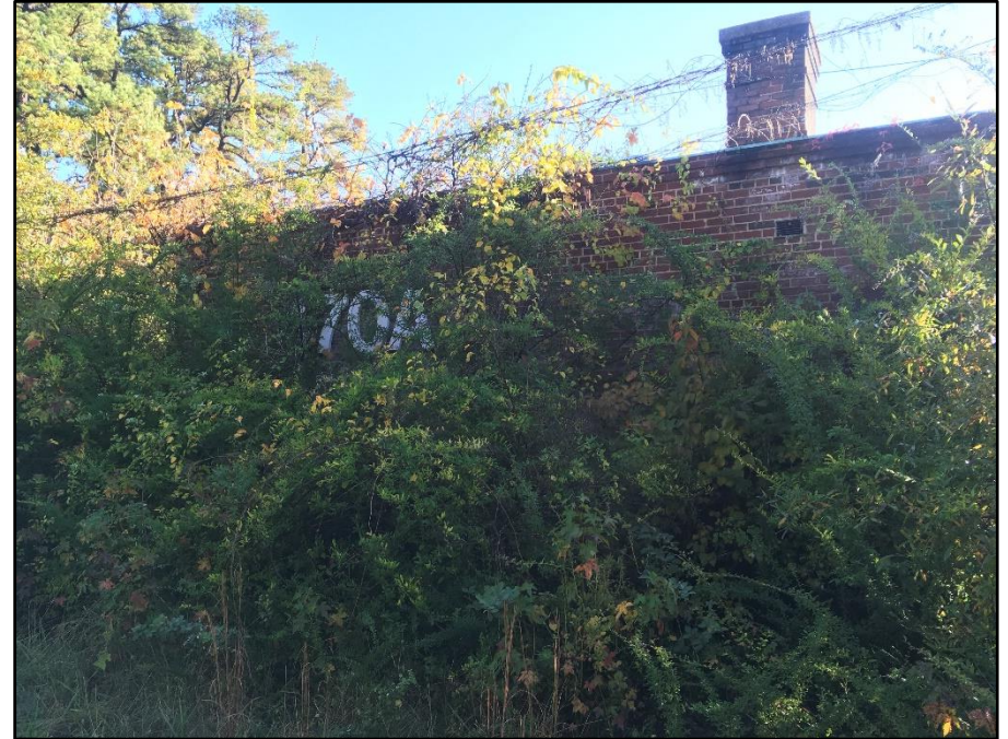
Photo 23: Building 470A, north side
