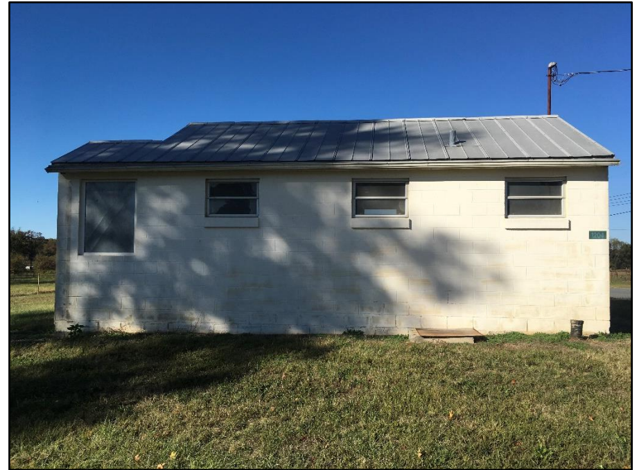
Photo 42: Building 1204, south side
