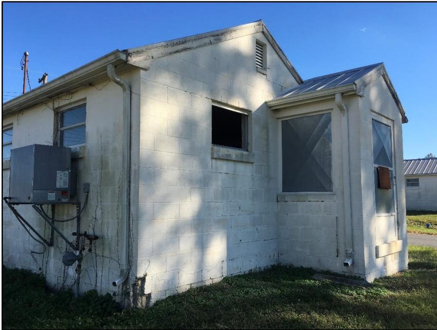
Photo 43: Building 1204, west (back) side
