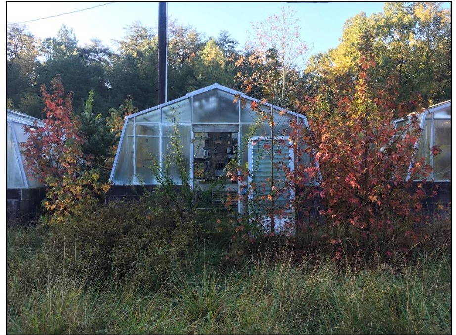
Photo 30: Building 470HH, north side (front)
