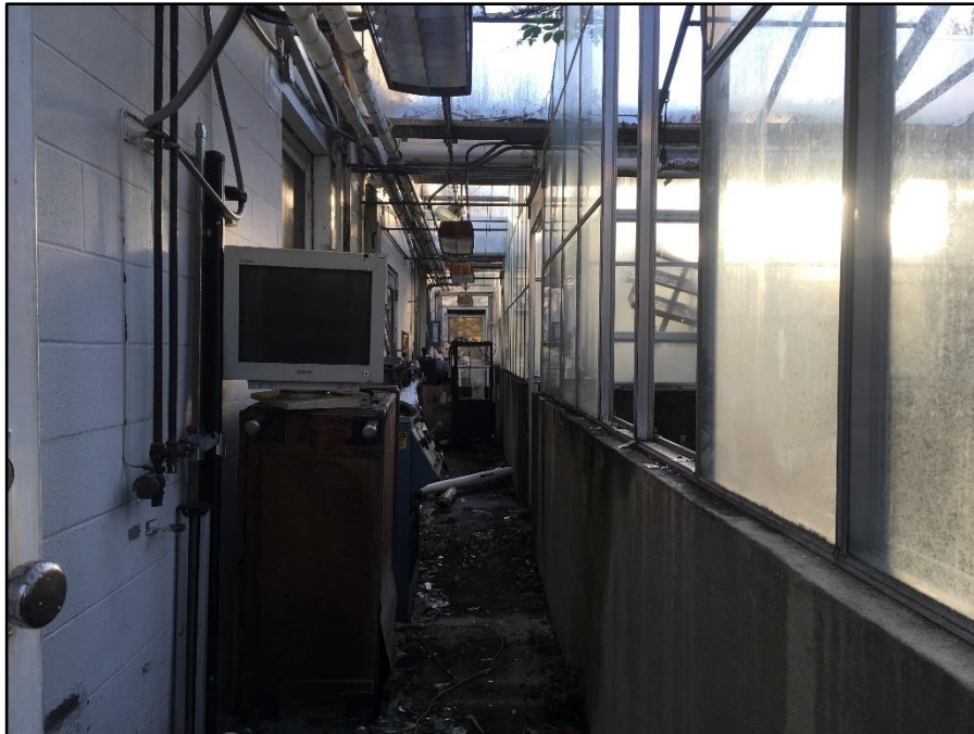
Photo 20: Building 465, inside of hall between main building and greenhouses
