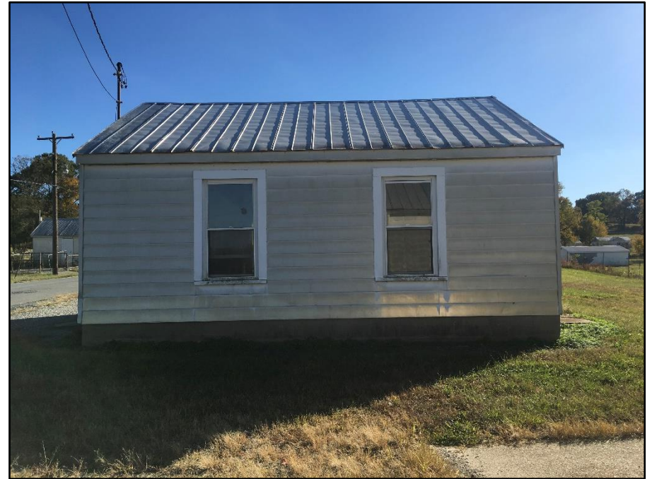
Photo 46: Building 1206, north side
