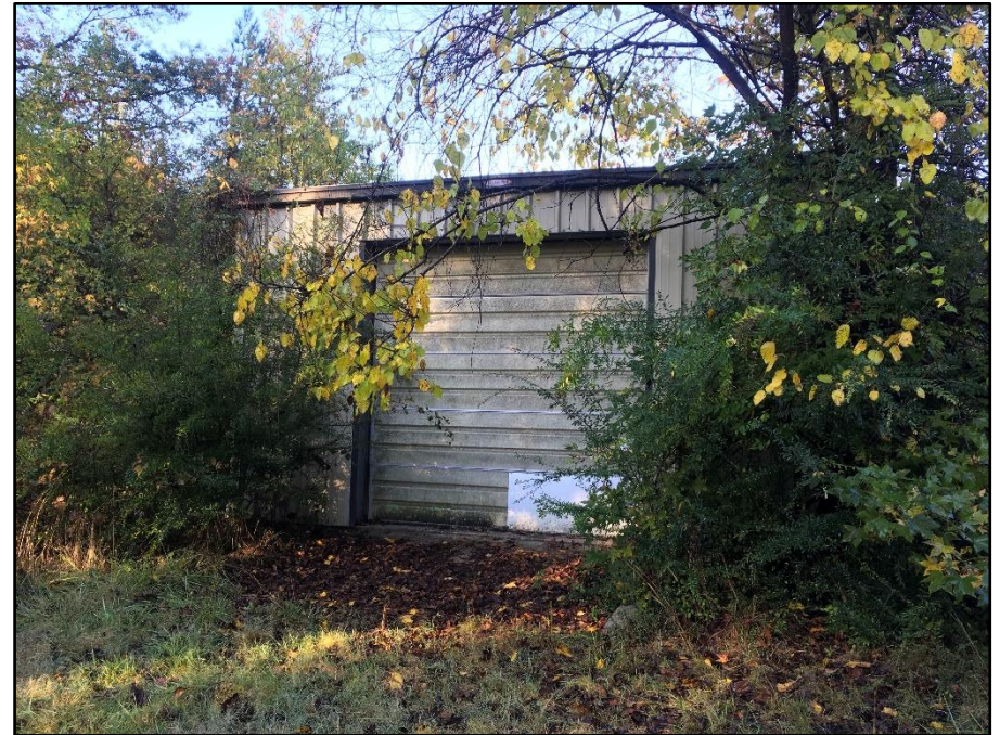
Photo 27: Building 470C, east side (front)
