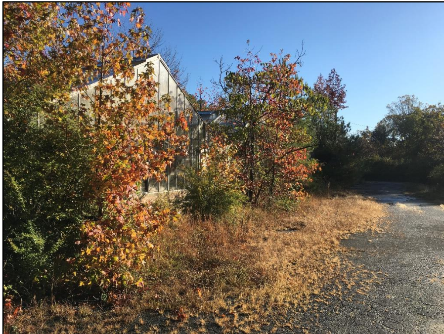
Photo 24: Building 470A, greenhouses attached at south side (back)
