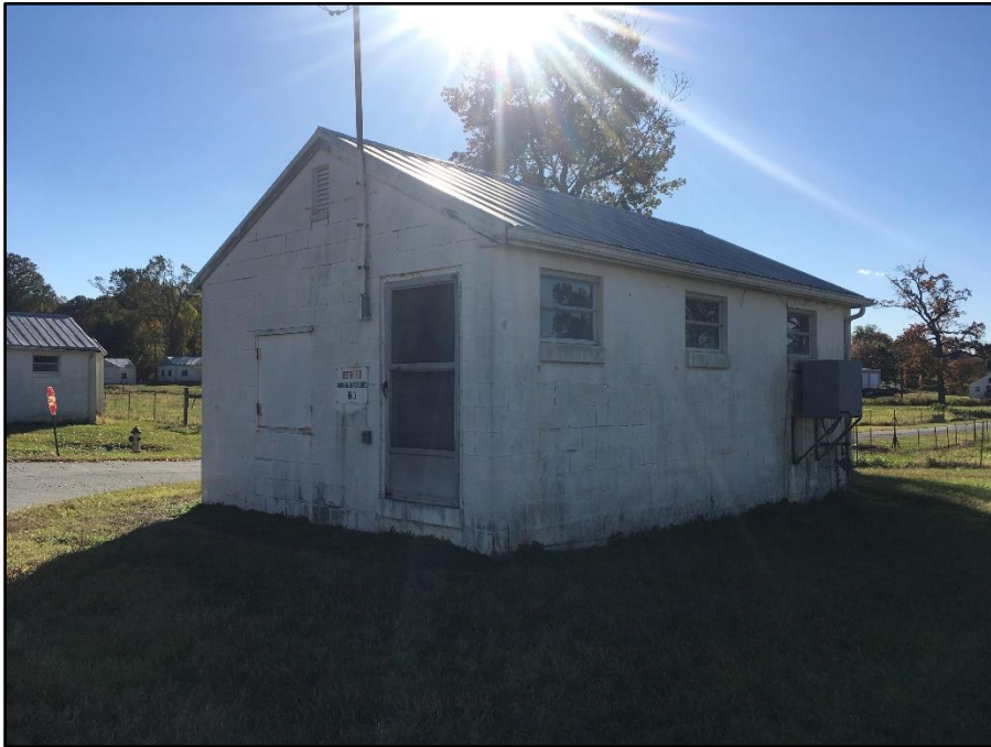
Photo 41: Building 1204, east (front) and north sides
