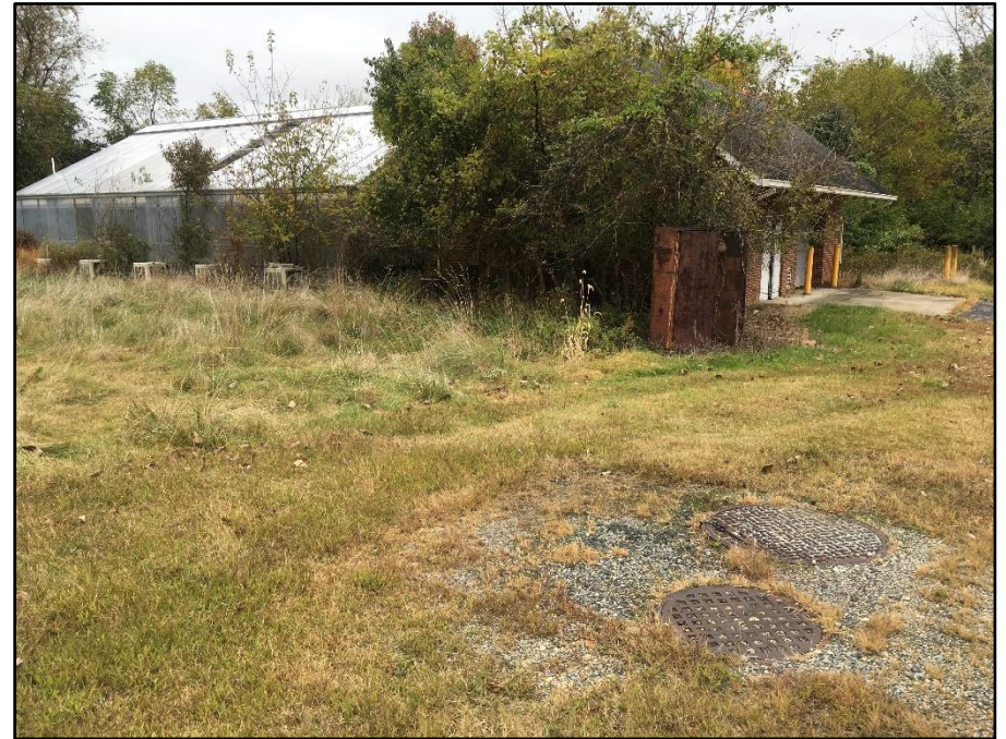
Photo 02: Building 053, west side and attached greenhouse at back
