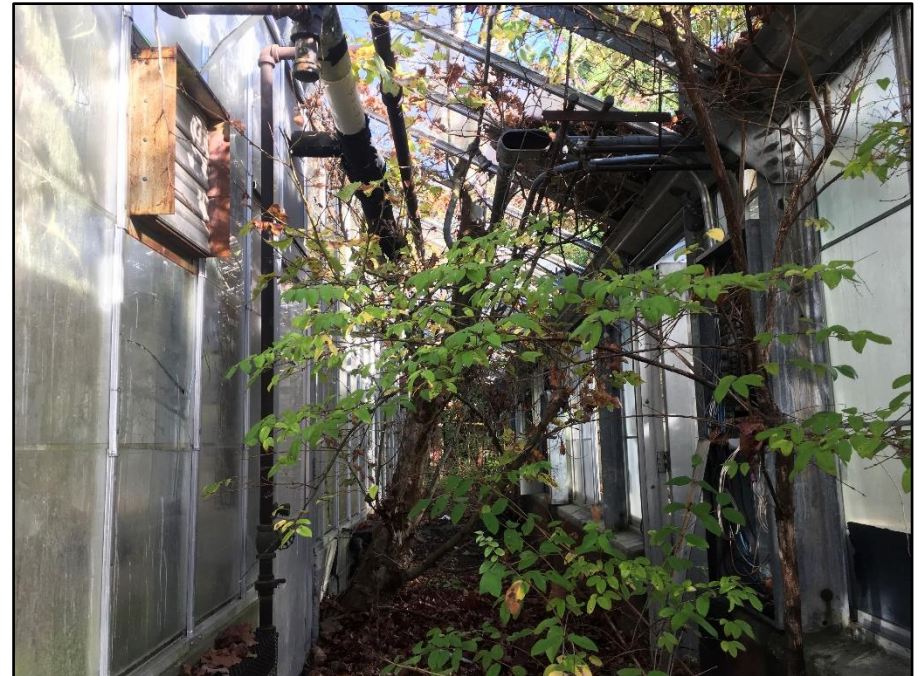
Photo 25: Building 470A, inside of greenhouse
