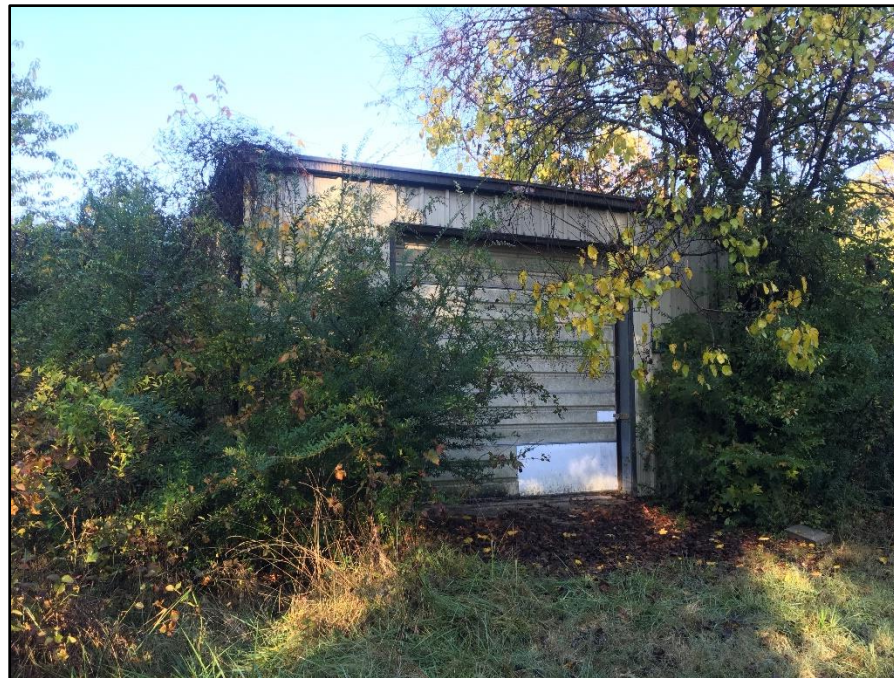
Photo 28: Building 470C, east side (front)
