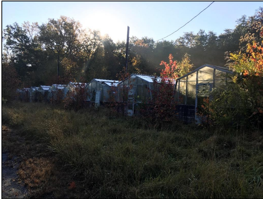
Photo 29: Buildings 470AA – 470JJ, north side (front) of greenhouses
